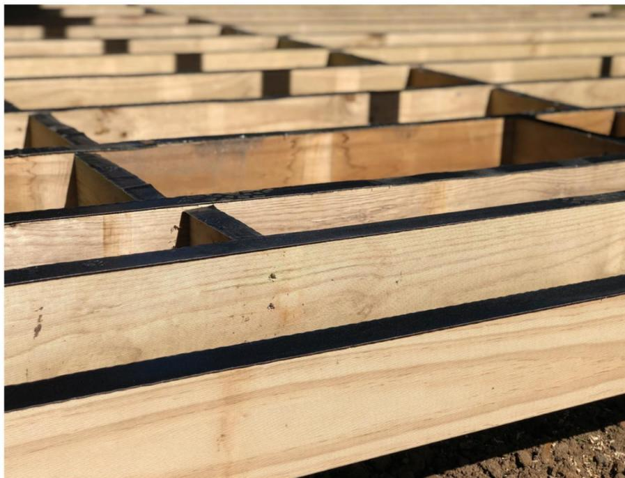
**ENGINEERED** with an aluminum liner, wider deck flashing tapes such as Trex Seal are available in widths from 11" to 22" to cover the entire surface of the ledger board—both on top and beneath—creating a seamless seal between the ledger, substructure and housewrap for optimal protection from water penetration.
