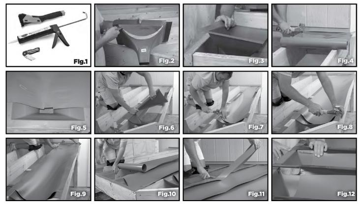
IMPORTANT: Water test prior to installation of decking and again after decking is installed.
